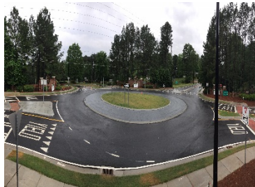
Road Construction $9.9M
