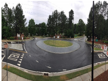
Road Construction $18.9M
