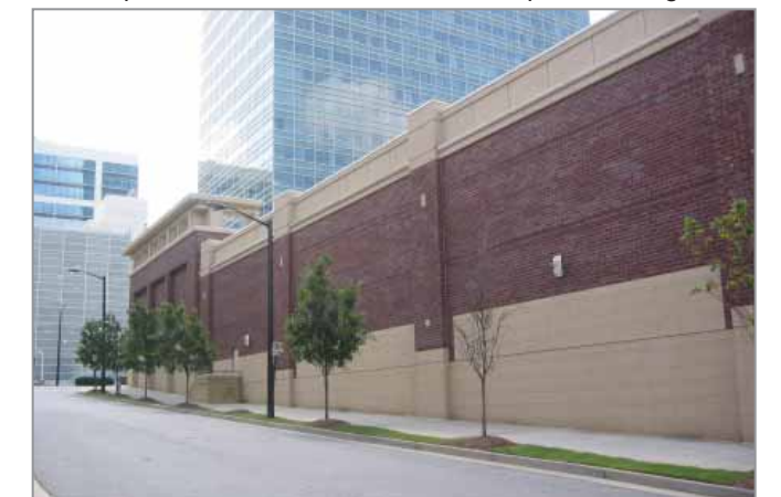
✗ Windows shall be a minimum of 15 percent of the total surface wall area along facades that do not face streets (excluding outbuildings).
