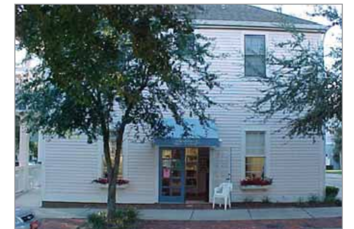
✗ All enfronting facades serving commercial uses: A minimum of 75 percent of the length of the enfronted portion of the build-to line shall be provided in glass.
