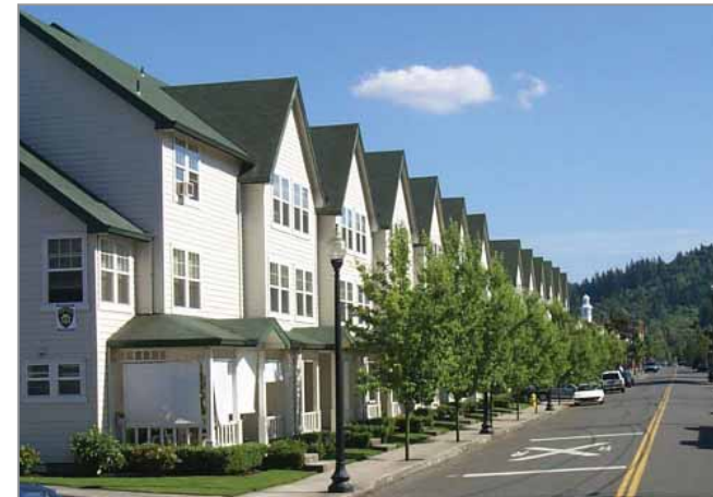
✗ Repetitive roof forms create a monotonous community in terms of design
