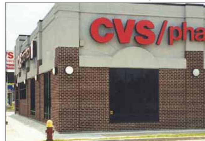
✗ Painted window or door glass is prohibited.
