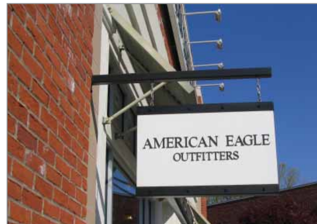
One blade sign for each business may be permanently installed perpendicular to the facade
