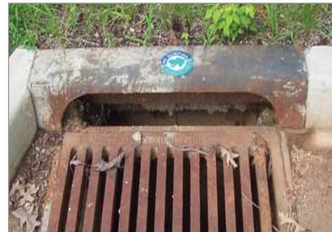
✓ Stenciling raises awareness of the materials that should not enter the storm drain.
