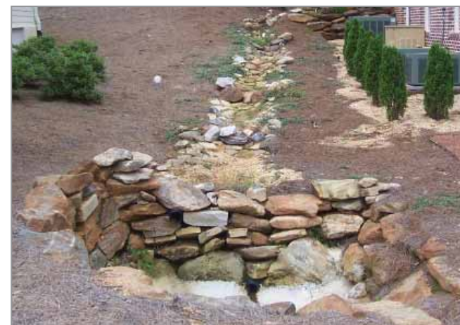
✓ Rocks or stones are recommended for stormwater drainage.
