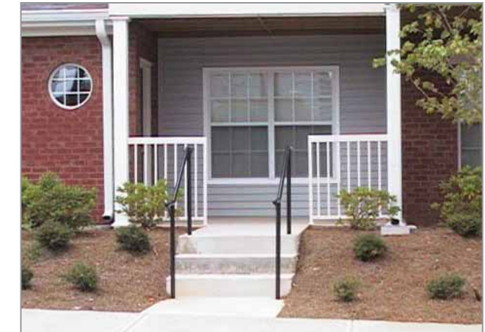
✗ A few steps are enough to make this entrance inaccessible to person with disabilities
