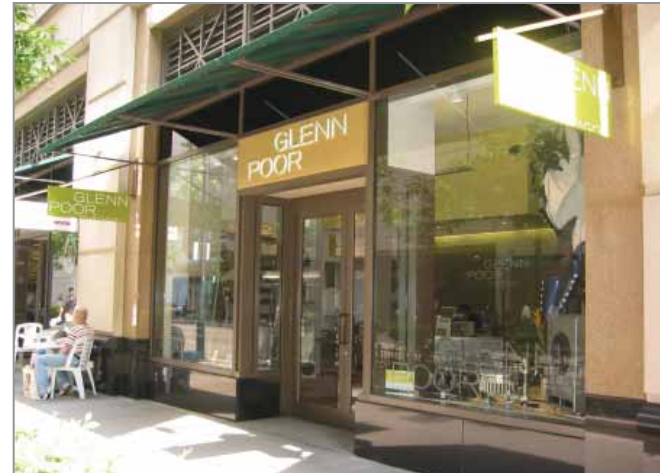
✓ Shopfront and Awning
