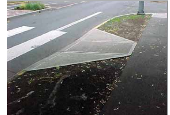
Ramps shall not exceed a 1:12 slope.
