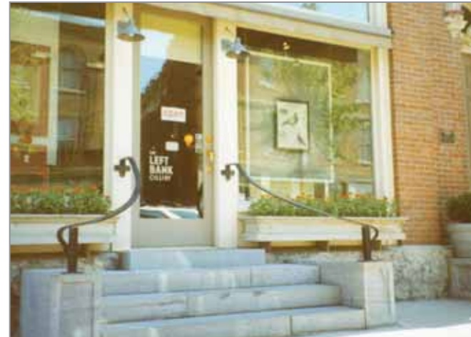
✗ Steps make visitability difficult on this business front door
