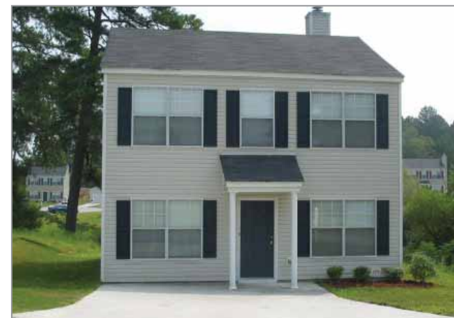
✗ Windows shall be square or vertical in proportion. Provide openings above the first story that do not exceed 50 percent of the total building wall area.
