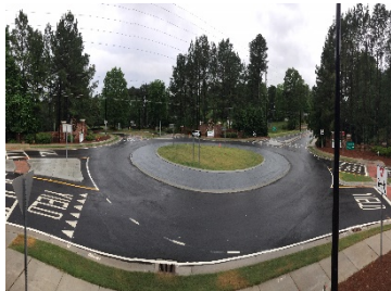
Road Construction $9.1M
