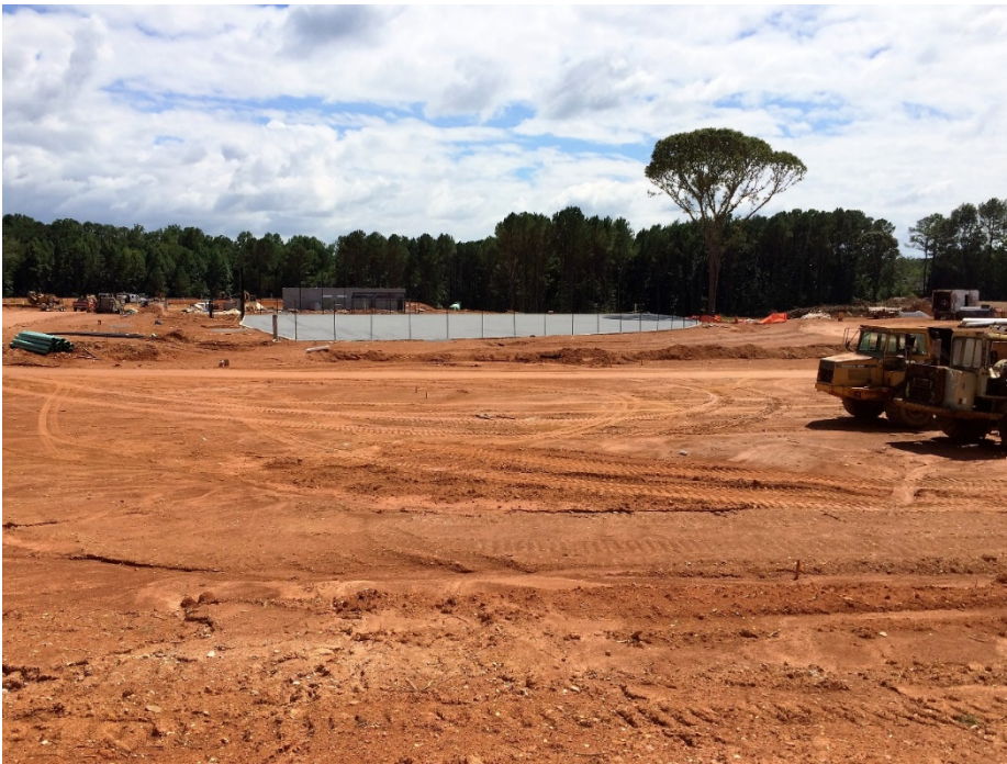
Site work in progress.
