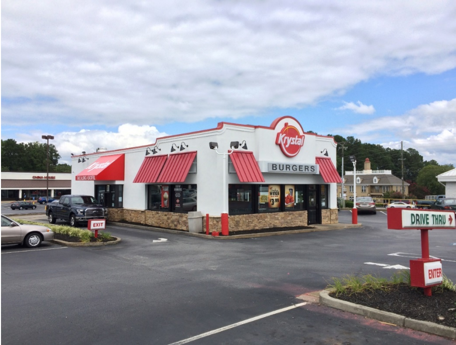
Façade and site improvements.
