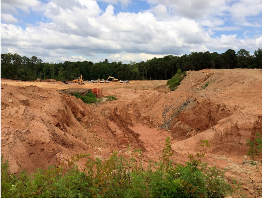
Site work in progress.
