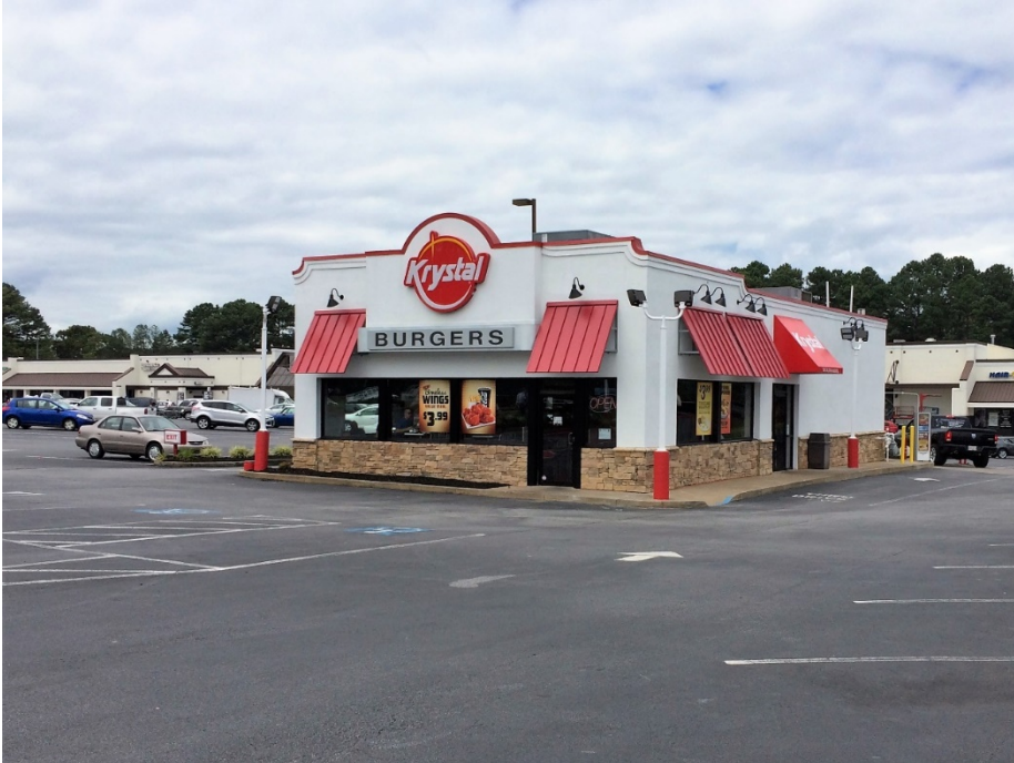
Façade and site improvements.
