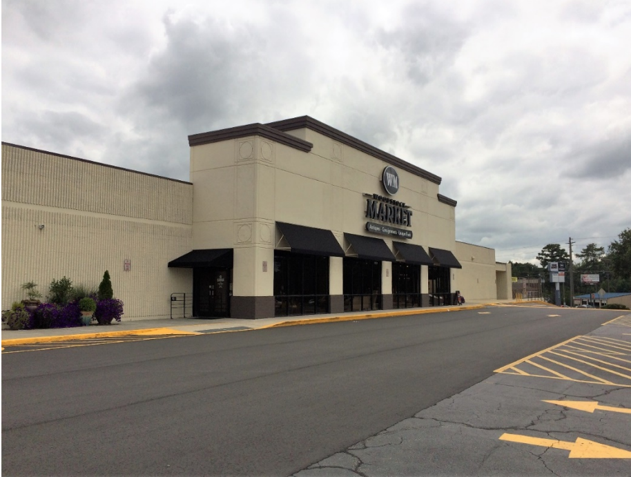
Woodstock Market – façade improvements.
