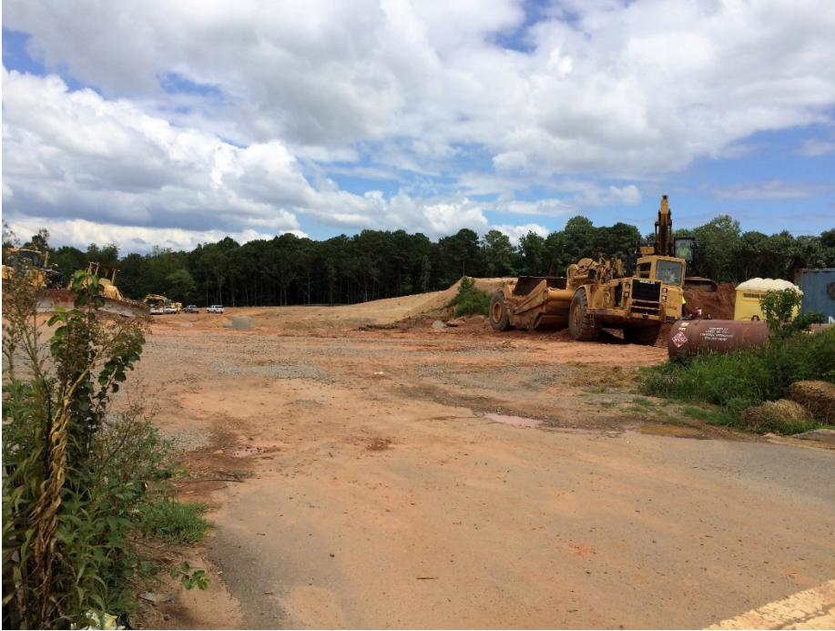
Site work in progress.
