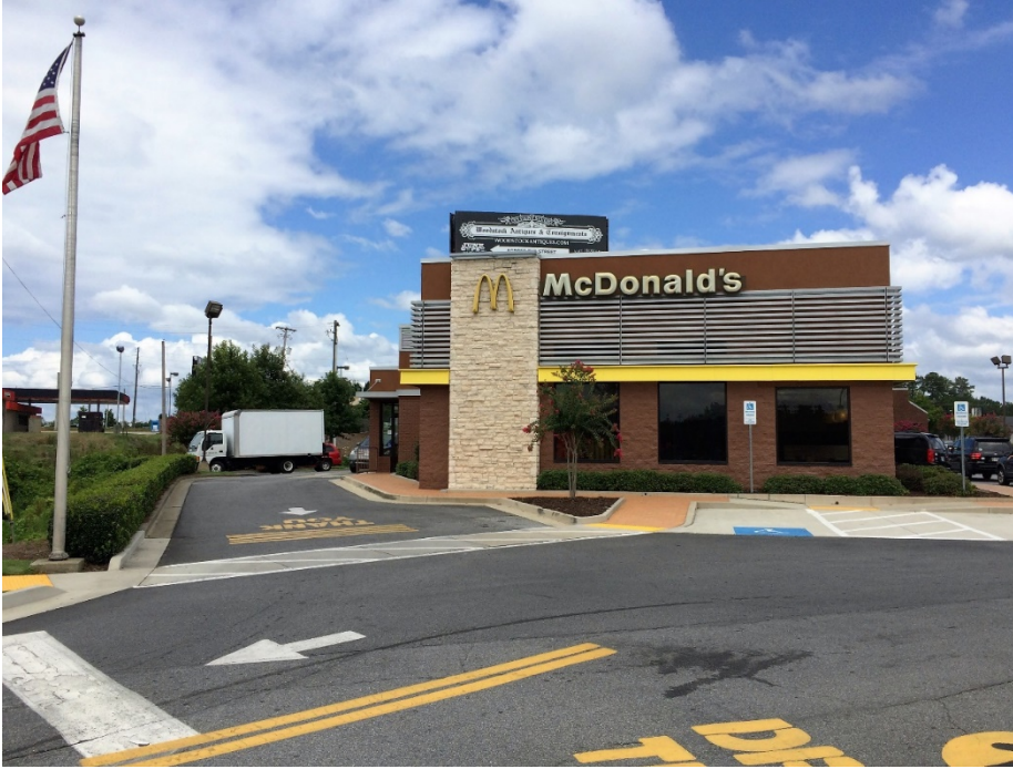
Façade and site improvements.
