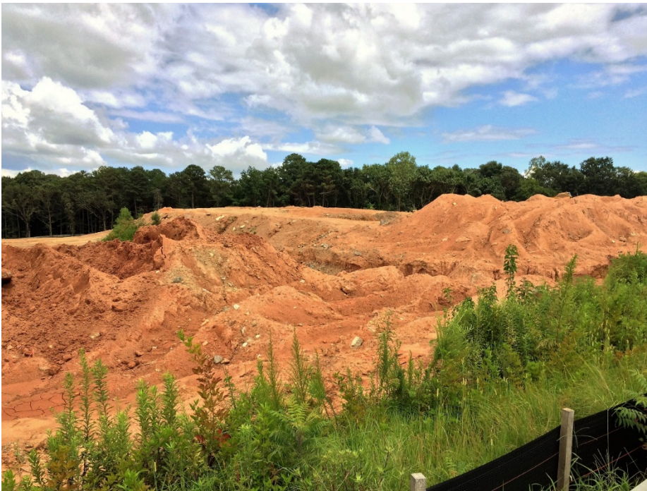
Site work in progress.
