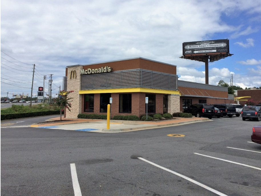
Façade and site improvements.
