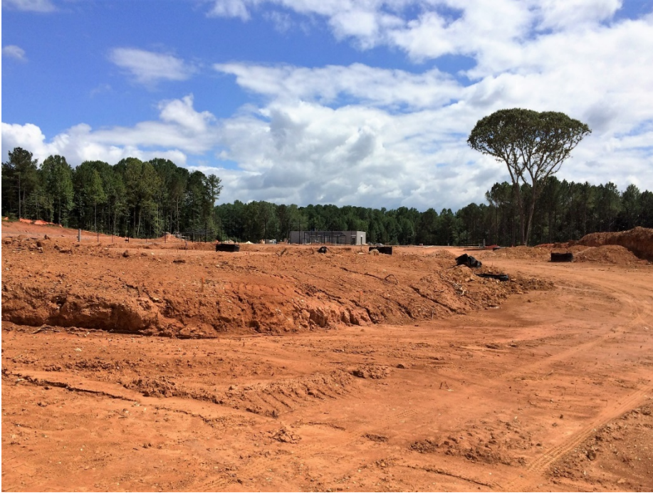
Site work in progress.
